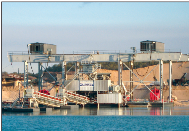
Coram's Supreme Manufacturing twin 13-yard dredge in full operation (above, left). Once material is processed, it's delivered to the plant's main separator the lake to approximately 300 acres," Vigliarolo told NAQN. "We are currently about one-fourth of the way finished with that and things are going very smoothly."
