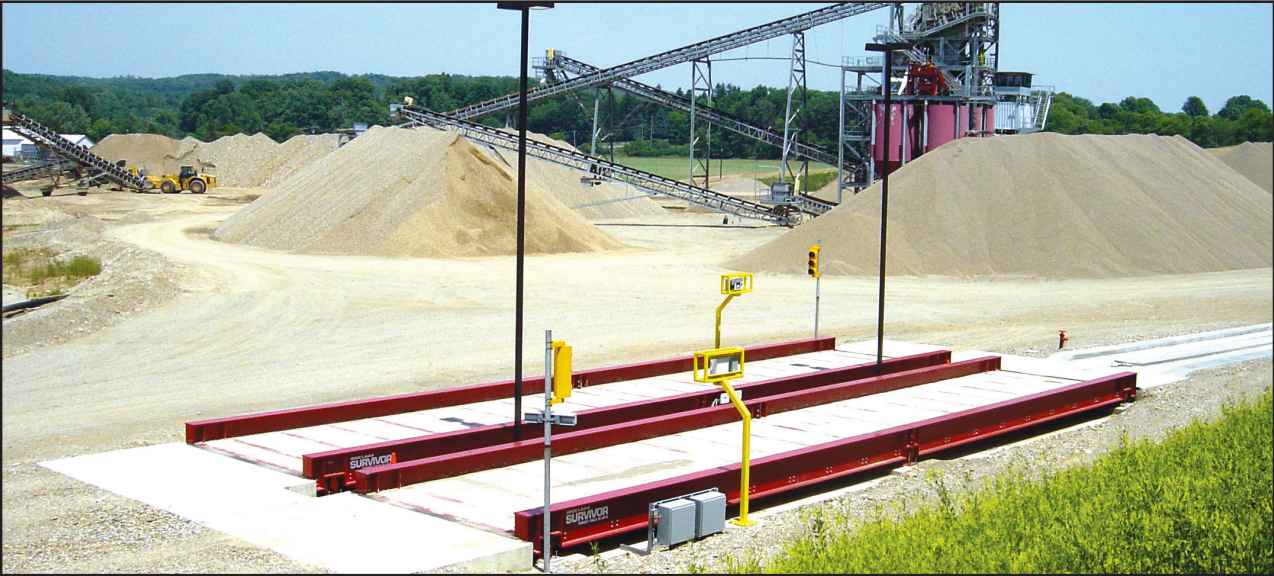
Inbound and outbound scales with computerized card readers, make customer visits to pick up material, quick and easy. Note the tire washing system on the outbound scale (right), used to clean the equipment before crossing the scale.
