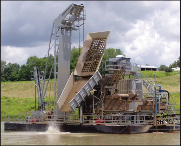
Deister screens work to size aggregate mined with the dredge.
