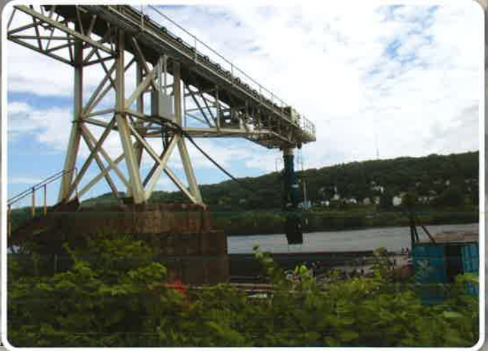
BARGE LOADING CONVEYOR
