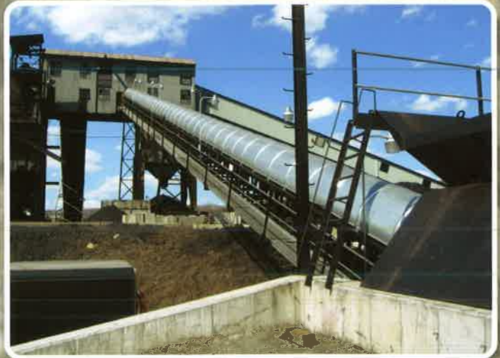
HOPPER & INCLINE CONVEYOR
