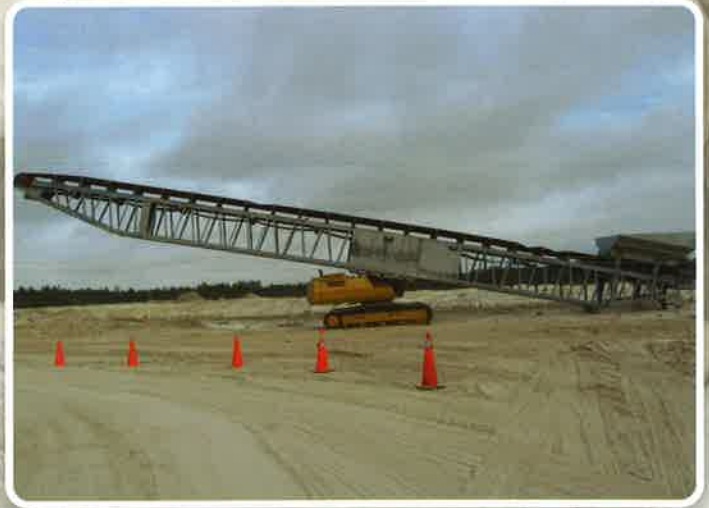
EXCAVATOR MOUNTED STACKER
