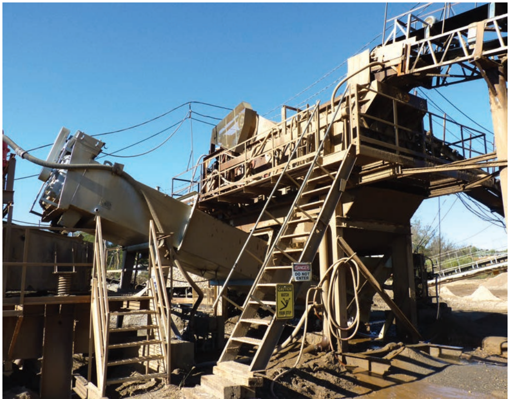
Material from the dredge passes through a triple deck Deister screen before going through an Eagle Iron Works log washer.
