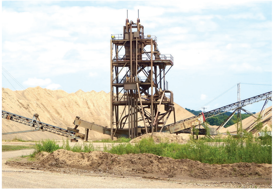
Material passes through the CFS tower where the Eagle Iron Works sand screws finish the dewatering job.
